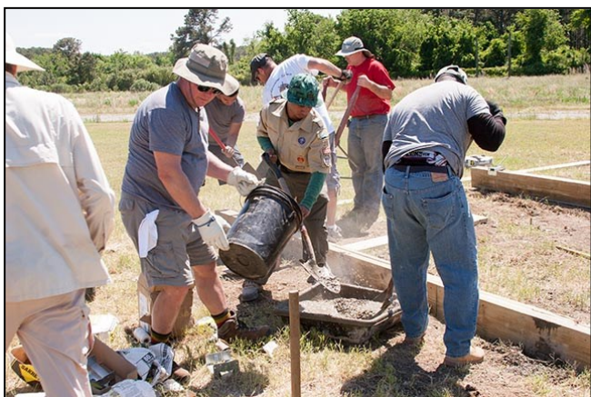
Kyle showing how to properly mix concrete for the footings.
