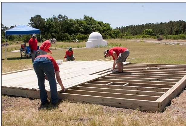
End of Day Two: footings, beams, joists and the first quarter of the decking complete. Notice the pier locations. The GAP POD is in the background.
